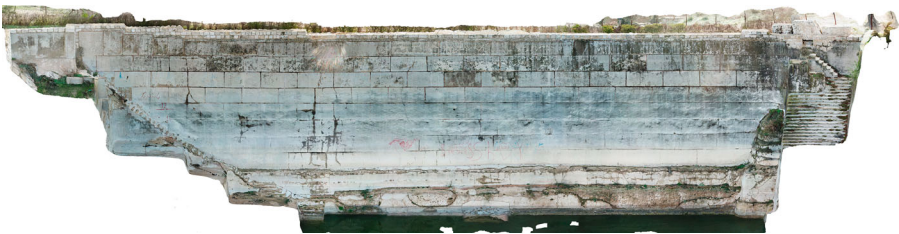
Figure 16. Orthophoto of the interior face of the Dam Wall, facing east.
