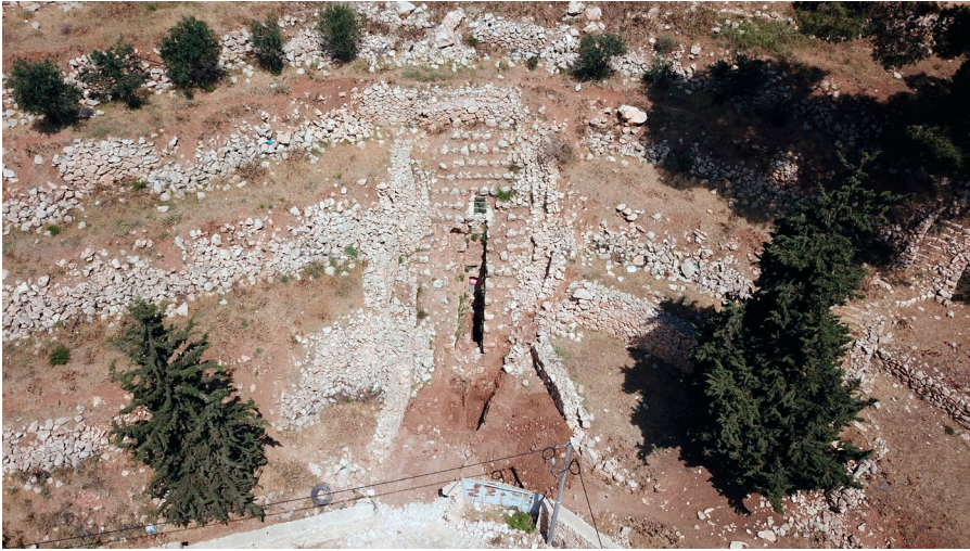
Figure 17. Photo of the Dam exterior from the east. The central opening through the stepped buttress providing access to the Dam interior is surrounded on both sides by modern agricultural terracing.
