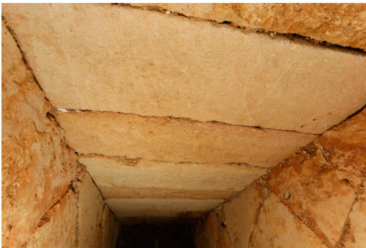
Figure 24. Photo of the ceiling blocks within the Dam staircase.
