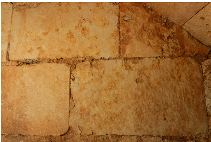
Figure 25. Photo of the wall blocks within the Dam staircase.
