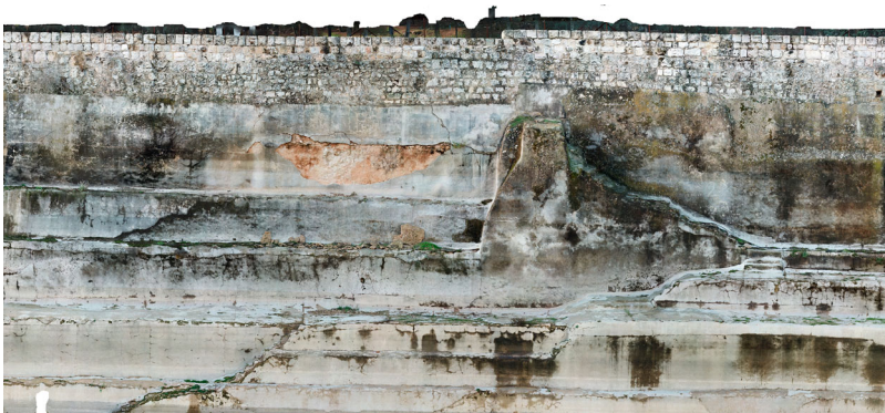
Figure 9. Orthophoto of the Southern Wall of the Lower Pool, showing collapsed plaster due to the buckling of the wall above. Collapsed plaster reveals bedrock with upper retaining wall. Note bedrock staircase cut off at centre right. The upper two courses of wall are of relatively recent vintage (ca. Medieval-modern).
